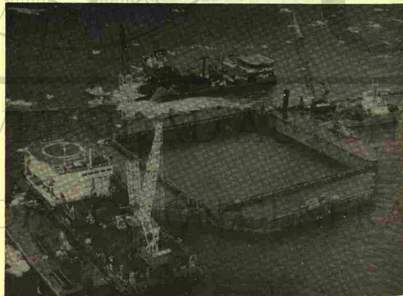
Fig. 10. Concrete Retaining Wall Caissins (14)
